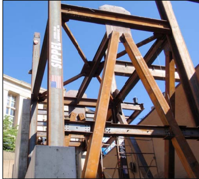
Figure 1 Structural Steel Braced Frame
