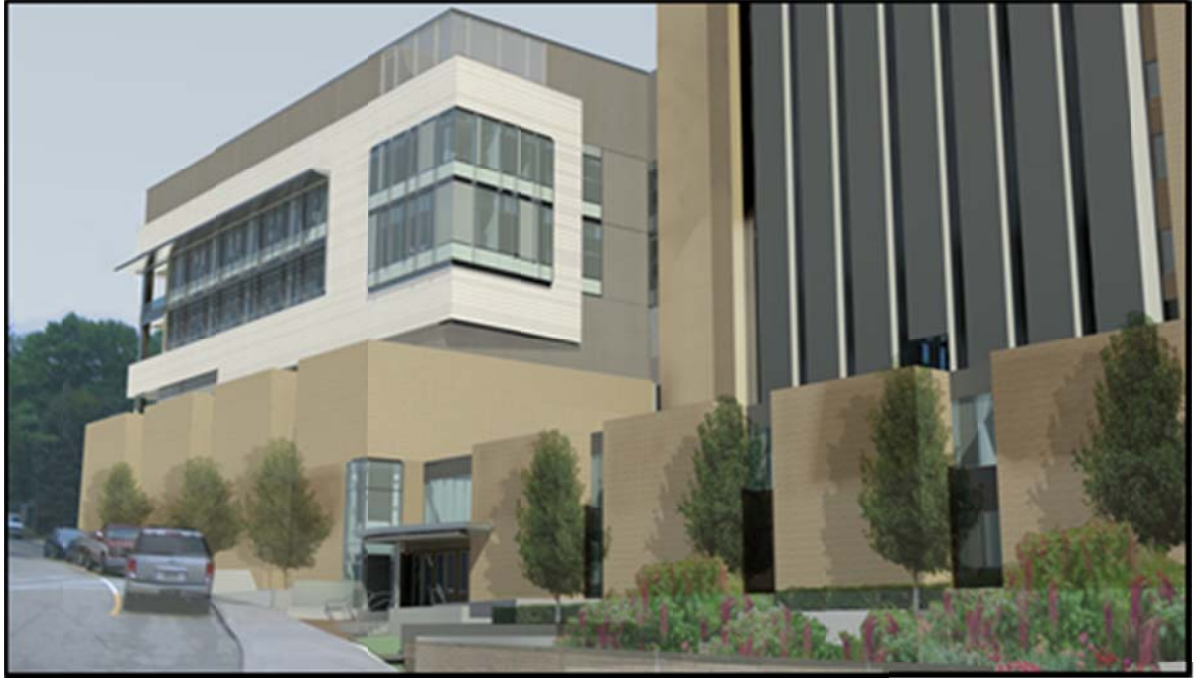
Photo Courtesy of Burchick Construction
