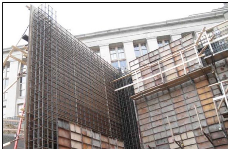
Figure 2 Rebar & Formwork for Concrete Wall at Generator Room
