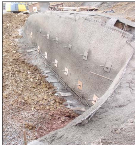
Figure 6 Soil Nail and Shotcrete
