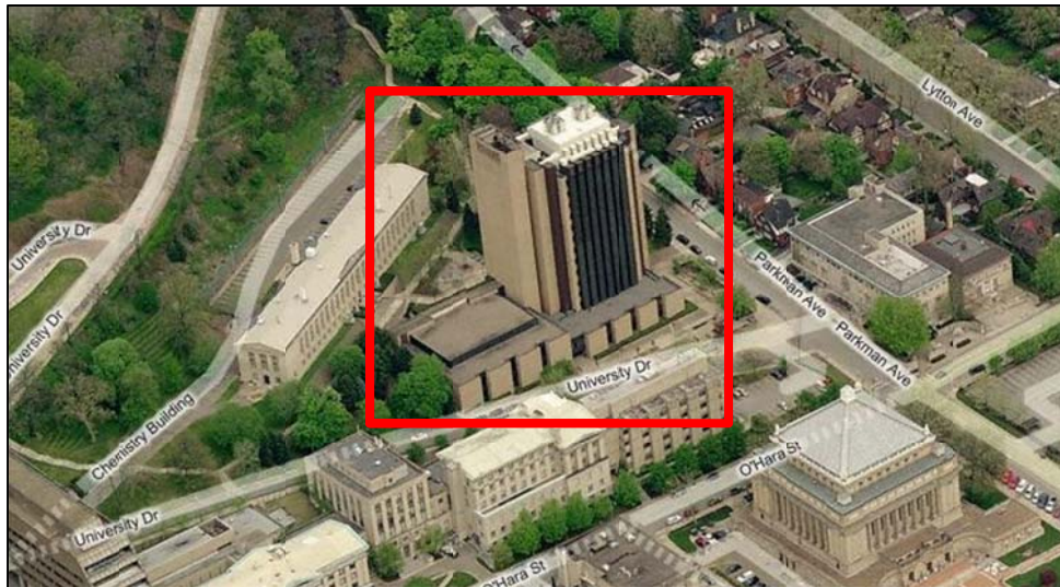
Figure 9 Bird's Eye View of the Chevron Annex and adjacent structures prior to construction
